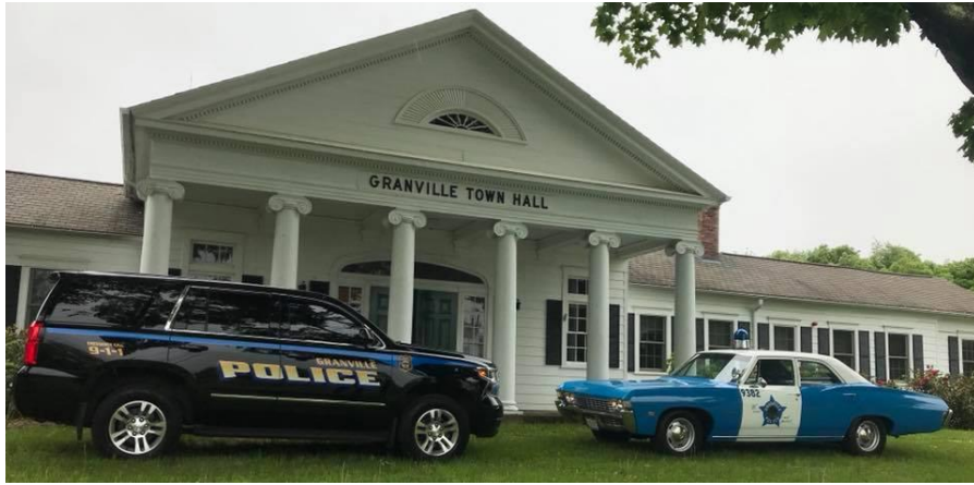
Figure 3-1. Granville Town Hall (Granville Police Department, 2020)
