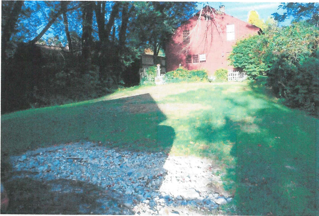
View east in the backyard where the replacement septic system is proposed: This location is 175 feet from the top of bank and at the outer limits of the 100-Year Flood Area.
